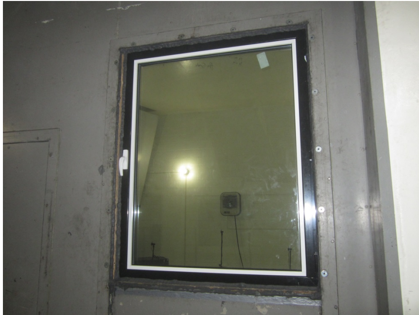
Receive Room View of Installed Test Specimen
